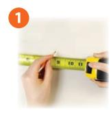
Determine first upright position. Then measure subsequent centers and mark
