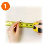
Determine first upright position. Then measure subsequent centers and mark
